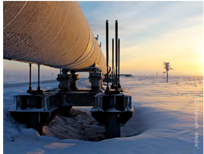
Our products and services help Velesstroy protect structures in harsh environments
