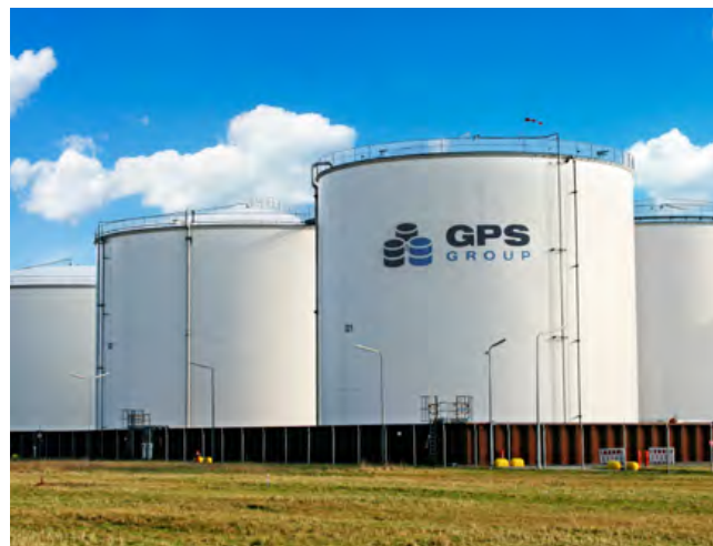
These petrol storage tanks in the Netherlands were repaired in just five months, without any asset downtime
