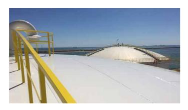
Our products have successfully protected the other 48 tanks at the terminal since it was constructed in the 1990s and we were asked to supply coatings for the  $20,000 \text{ m}^2$  of new steel.
